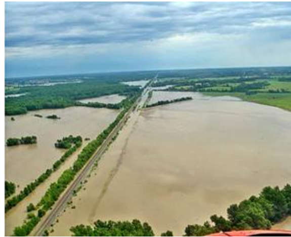
Aerial view of flooded railway.
